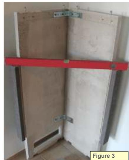
With turning the bottom screws with a 8er flat spanner, the chamotte side parts can be set to perpendicular and horizontal state (Figure 2 u. 3). The lower bracket can be tightened by hand right after the adjustment of the plates. If the plates are set perfectly, the F90 - fire protection plate can be pushed in the lower rabbet (Figure 4).
