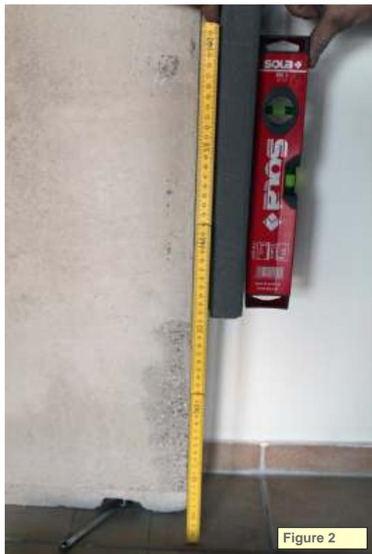
The next step includes the loose (!!!) mounting of the side plates. Please connect the plates at the designated spots with the delivered brackets and thumbscrews, flat washers and retaining rings. The adjustment of the walls is done by regulating the distance between the rabbet of the side wall and the ground to 30.8 cm (Figure 2).
